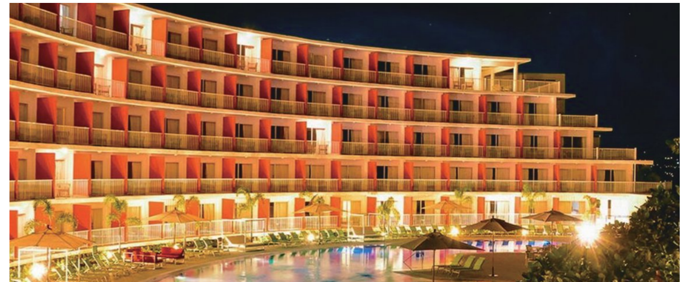
Montego bay resort in Jamaica, with DC inverter VRF system.
