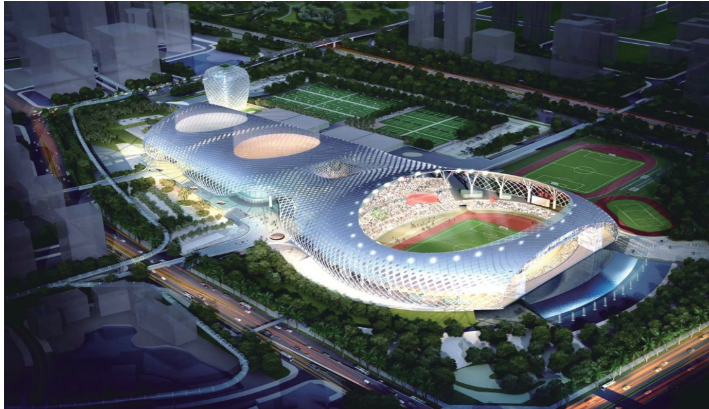
Main venue of the Universiade in Shenzhen, total VRF capacity 8000 kW.
